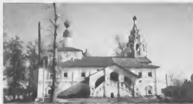
Fig. 14.224. The Church of Presentation, the Nikolo-Ouleimskiy Monastery, Ouglich. Northern view. The church is entered via a tall porch that leads directly to the first floor. Photograph taken in 2000.
